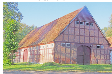
Farm house in Münsterland
